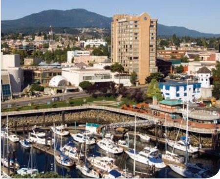
The Bastion (seen here on the right) defines the downtown harbour area (Terry Patterson, www.terrypattersonphotography.com )
